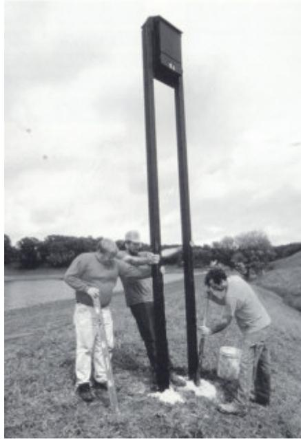
*Concrete can be mixed directly in the hole (use several bags of mix per hole). While mixing, check the poles frequently with a level to ensure they are vertical.*
