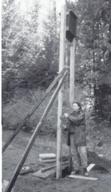
*Project Assistant Selena Kiser checks a pair of nursery houses with a level to ensure the poles are vertical. Temporary braces and stakes were used to hold poles in place while the concrete mix dried.*
